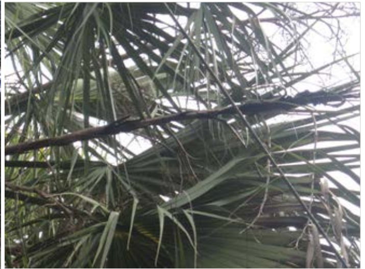
(SCE&G power line contacting palm fronds)
